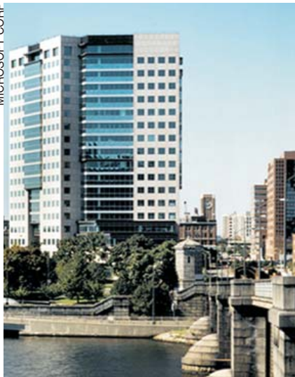
Microsoft Research New England will be housed in this building near the MIT campus.
